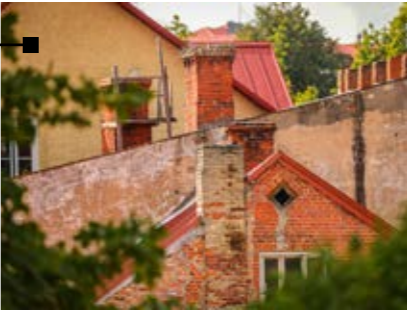
The roofs of the old town of Kandava
